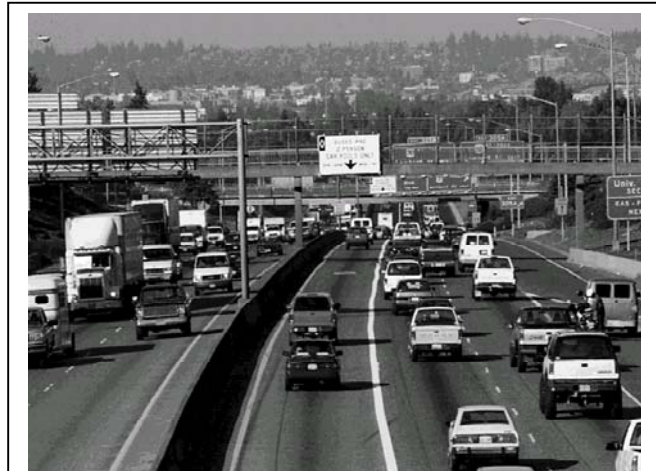
About 950 vehicles (2,450 people) daily use this high-occupancy vehicle (HOV) lane on northbound I-5 in Portland. During peak periods, car-poolers shave up to 20 minutes from their commute.
