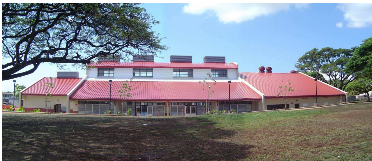
Figure 2.02 – North Elevation of the WIS Cafeteria as seen from Farrington Highway Sustainable design strategies that were used in obtaining the LEED Certified rating include:
