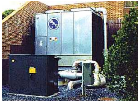
Figure 3.12 - Cooling Tower
