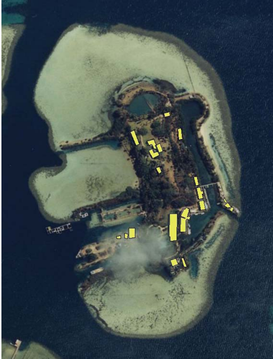
Figure 13 - Identified Rooftops of Coconut Island
