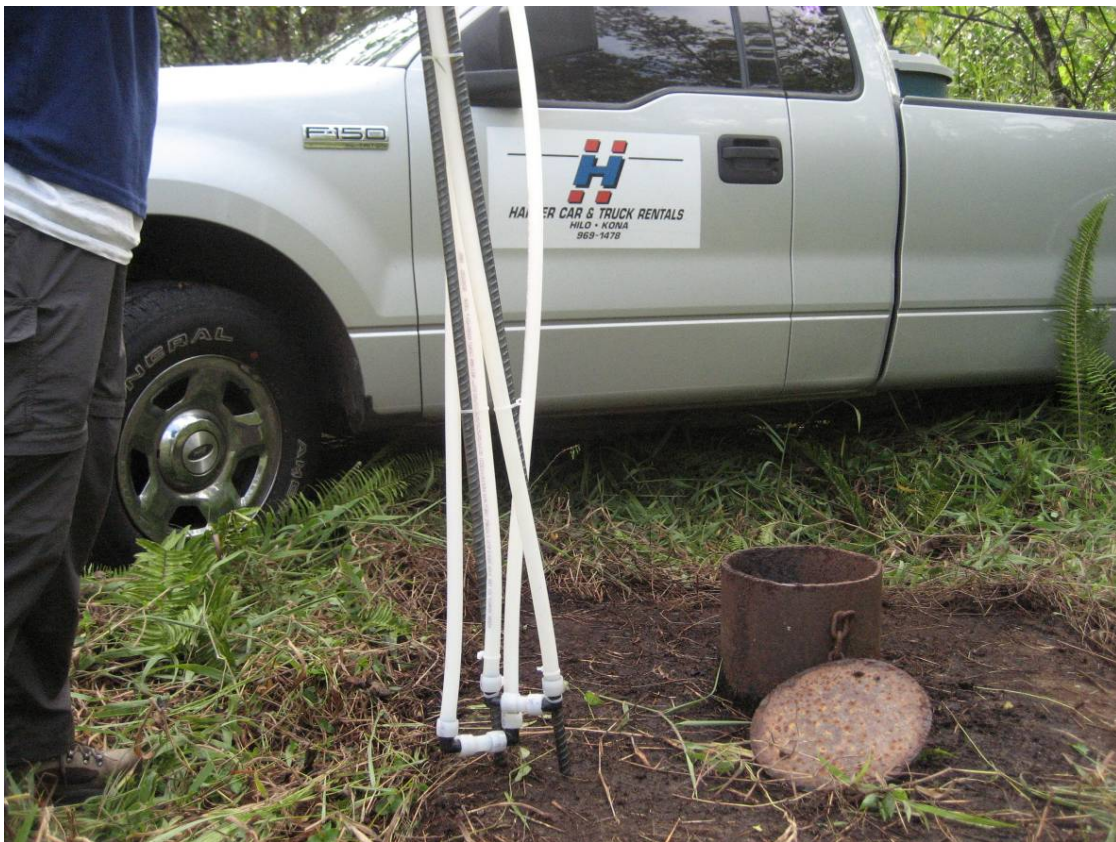
Figure 3. Photograph of the PEX DHE assembly prior to insertion into the Malama Ki well ( note rebar fastened to the PEX tubing and the well in the lower right-hand corner ).
