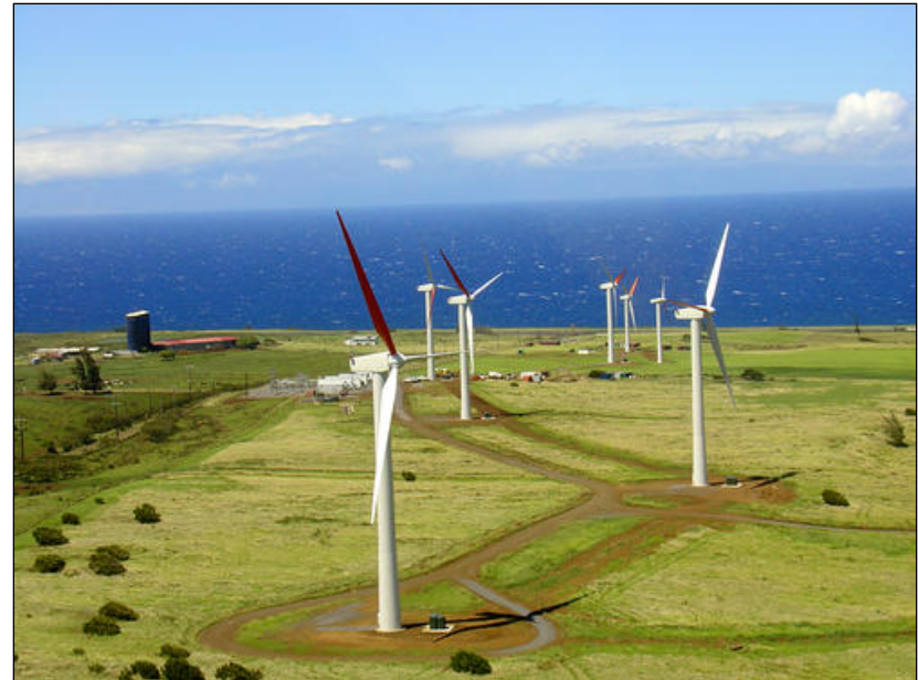
Hawi Renewable Development LLC Wind Farm at Upolu Point near Hawi on the Island of Hawaii. Source: Hawaiian Electric Light Company via NREL Photo Information Exchange.
