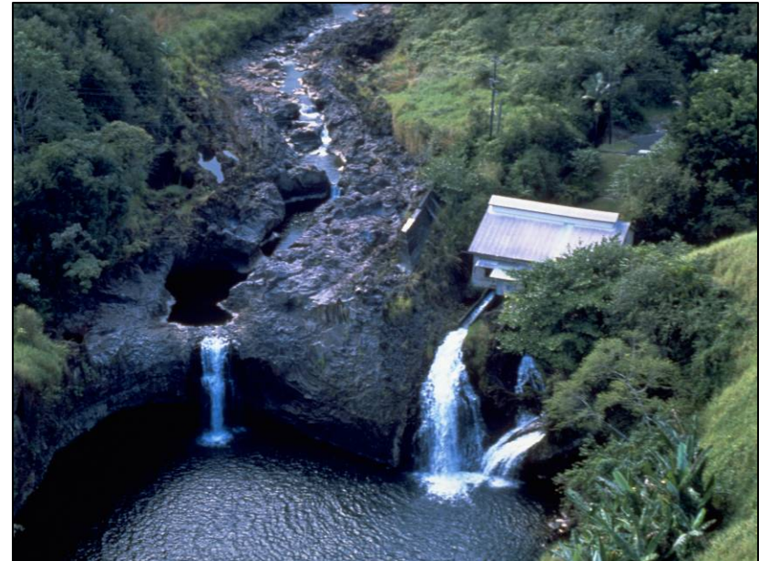
Waiiau Hydroelectric Plant, Wailuku River on the Island of Hawaii. Photo: HECO.
