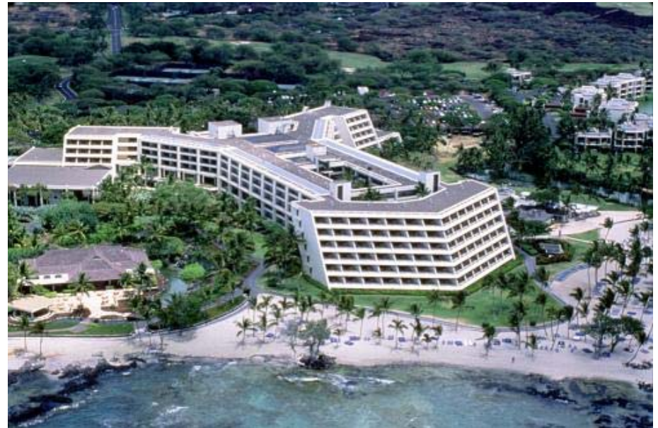
Mauna Lani Resort has 80 kW of Solar Panels on Roof and over 500 kW total on property on Island of Hawaii. (Photo: PowerLight)
