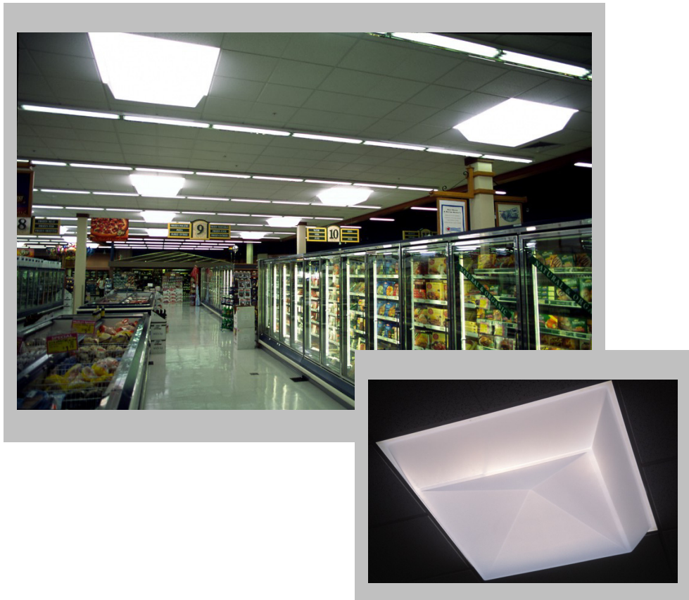
Figure 3-25. Foodland, Ewa, Oahu. Skylights and integrated light wells with diffusers (inset) at the ceiling. Photos: Erik Kolderup, Eley Associates.
