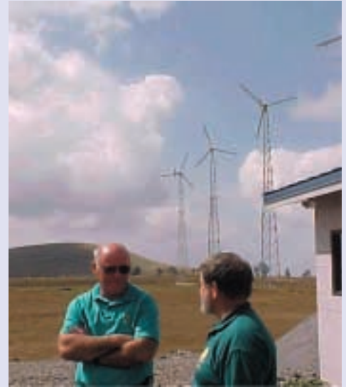
Frank Hess, Service Operations Manager, Parker Ranch (on the left) and John Crouch, Director, PowerLight Corporation , shown next to the control building, with three of the five 10 kW wind turbines in the background. The Supervisory Control and Data Acquisition (SCADA) system maximizes the efficiency of the hybrid system by matching electrical load to available solar energy.
