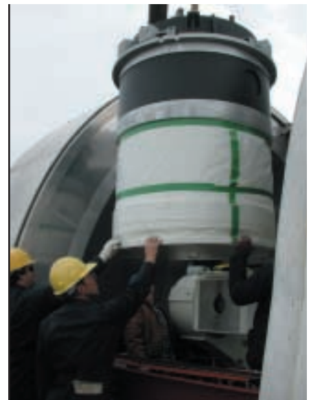
The U.S. Air Force (USAF) has begun improving its ability to track 500 deep-space satellites from atop Haleakala by refurbishing three telescopes at the Maui Space Surveillance Complex . Above, workers lower the 14,800-pound Ground Based Electro Optical Deep Space Surveillance System (GEODSS) telescope onto its new mount.
