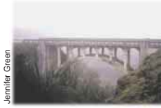
Dry Canyon Bridge
