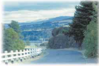
HCRH near Mosier Twin Tunnel
