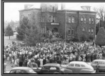
Polk County Courthouse Then
