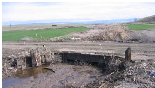
Sediment plugging up Gerking Creek (tributary to Wildhorse). Approximately 6' clearance under bridge.
