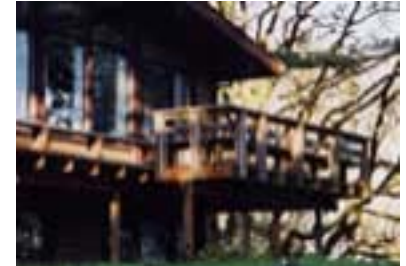
Residential wood decks will no longer be constructed with copper chromated arsenate (CCA) treated lumber.
