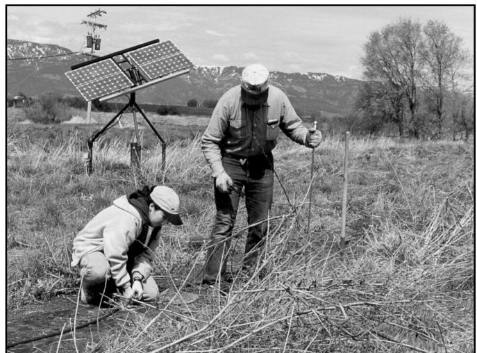
Photovoltaic-powered drip irrigation system
