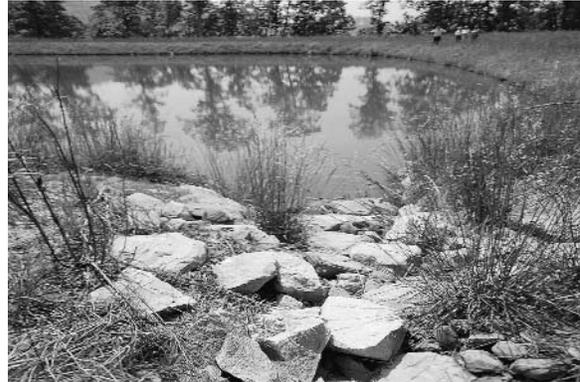
*Erosion controls such as sediment ponds prevent material from getting off the mine site. Photo Credit: Chuck Meyers, OSM*
