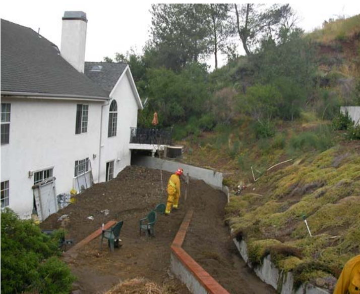
A house in Modjeska Canyon suffers damage from a debris flow on May 22, 2008. Photo courtesy Orange County Fire Authority.
