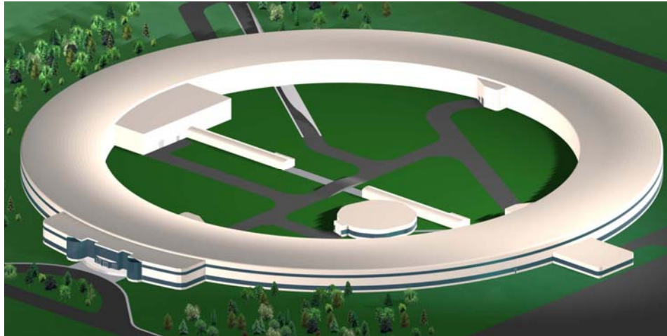
Figure 3.3.1 Computer rendering of the exterior of the NSLS-II storage ring. The main entrance is shown to the lower left, the RF gun chamber is to the lower right outside the ring, and the buildings housing the klystron galleries for the linac injection system (which is itself below ground), are shown in the infield of the ring. The small circular building in the infield is the IR ring, which shares the first portion of the same injection system used to top-off the X-ray ring.
