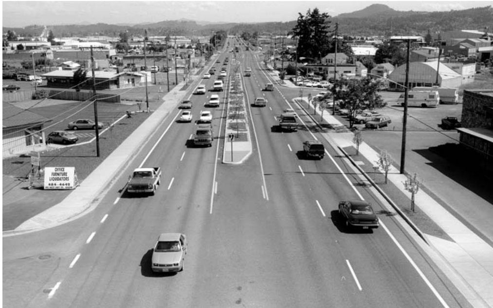
A nontraversable median with plantings on Pacific Highway West in Eugene.
