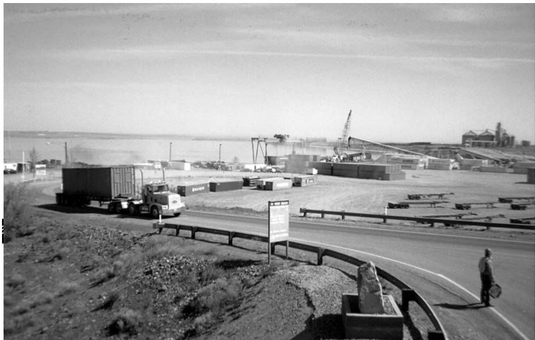
The intermodal connector at the Port of Morrow connects Interstate 84 to port facilities where goods are transferred from truck to barge. (Photo courtesy of Port of Morrow)
