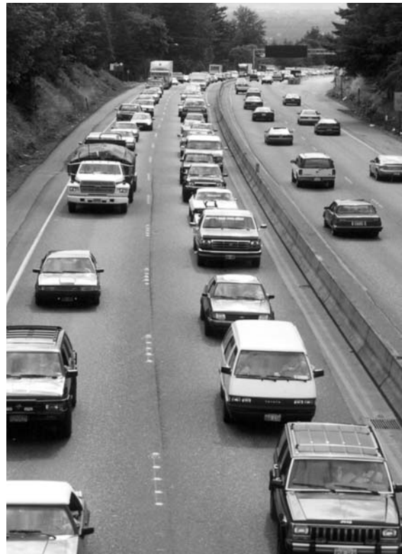
Traffic is bunching up and slowing down in all lanes of this freeway because traffic demand exceeds capacity.
