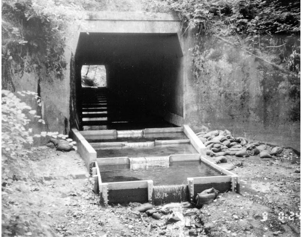
This retrofitted culvert has increased water depth, lower water velocities and a concentrated flow that will form a jump pool for endangered salmon in King Creek on the Coos Bay – Roseburg Highway (Oregon 42)
