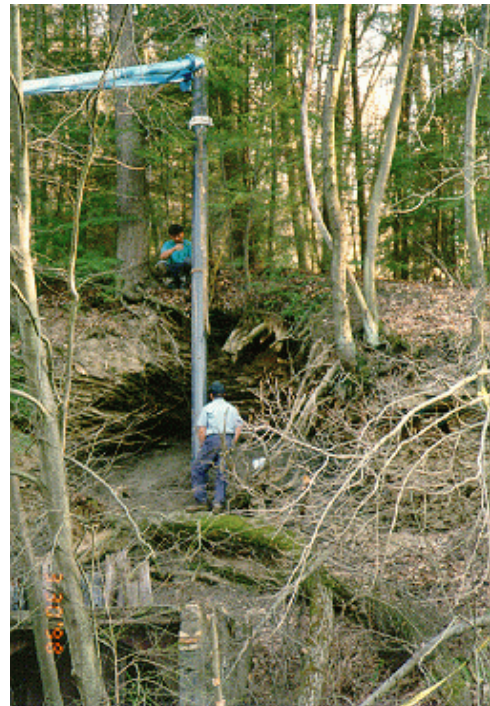
Figure 15 Installation of vent at gassy abandoned portal, entry backfilled with concrete.
