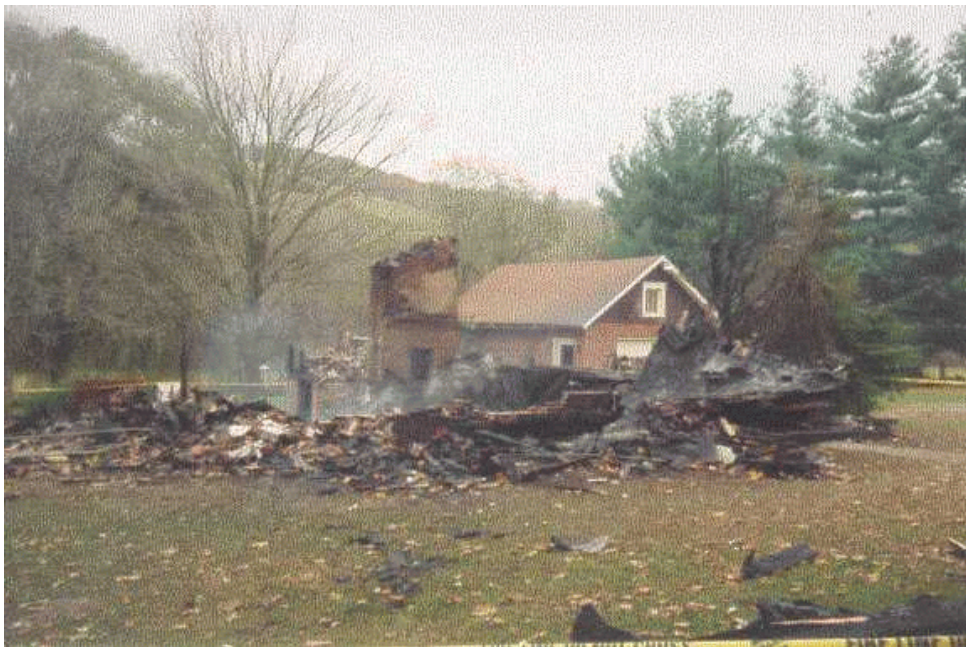
Figure 1. Remains of a two story residence as a result of an explosion from uncontrolled fugitive methane.
