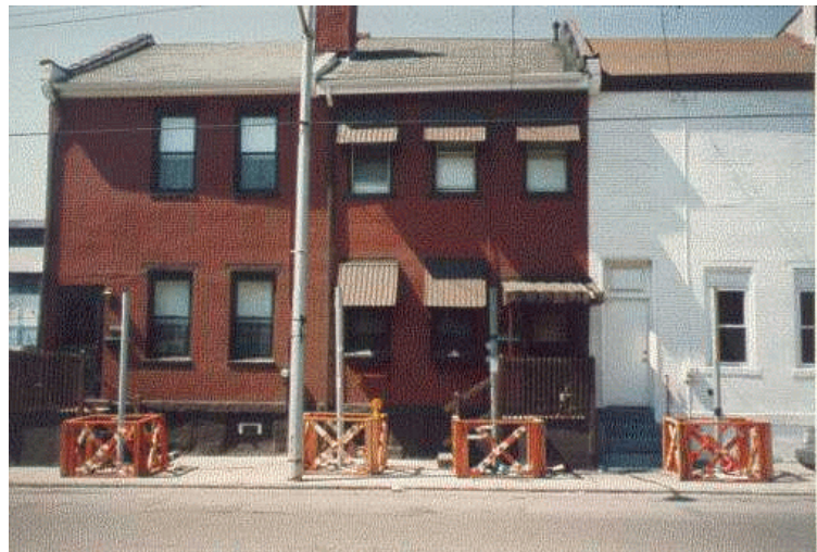
Figure 22. Vent stacks outside of residential structures.
