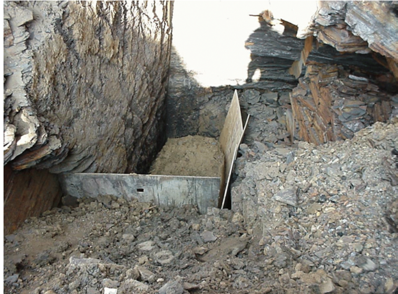
Figure 24 Soil-Bentonite cut-off trench excavated into collapsed mine voids. (OSM-FRPD)
