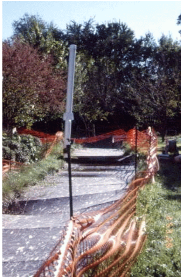
Figure 19. Water well vent.
