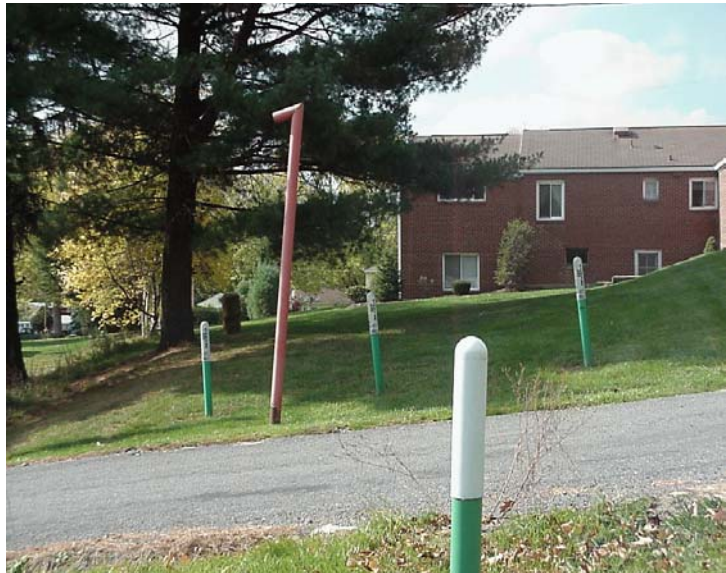
Figure 21 Red gas vent along gas pipeline right of way is used to safely conduct gas from a shallow mine subsidence. (OSM-FRPD)
