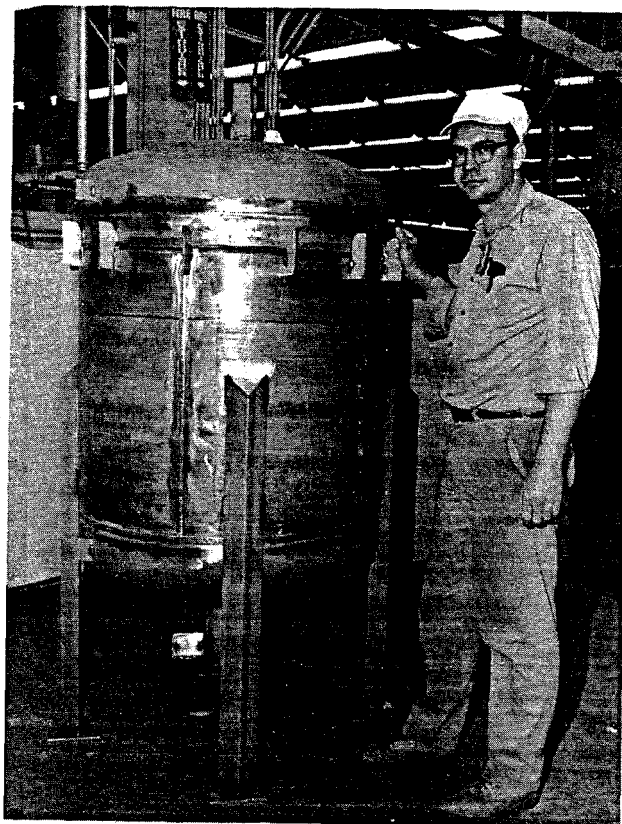
Pressure vessel being fabricated in Central Mechanical Shop, Building 7012. Gary Petrey, boilermaker, is shown beside the pressure vessel (1977). ▶
