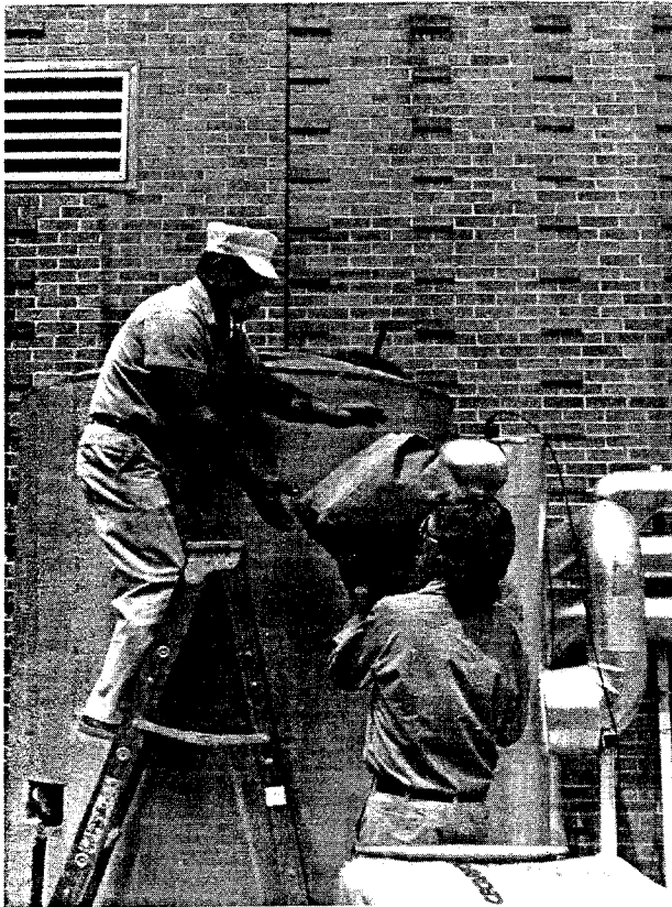
▲ Maintenance of charcoal filters (replacing charcoal) that remove chlorine from process water used in aquatic experiments (Aquatic Laboratory, Building 1504). Bruce Bennett (left) and LeRoy West (1990).
