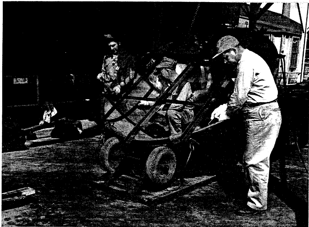
Leadburners fabricating sulphuric acid vat. C. W. Wright, P. E. Hornsby, and W. C. Garrison (1951). ▼
