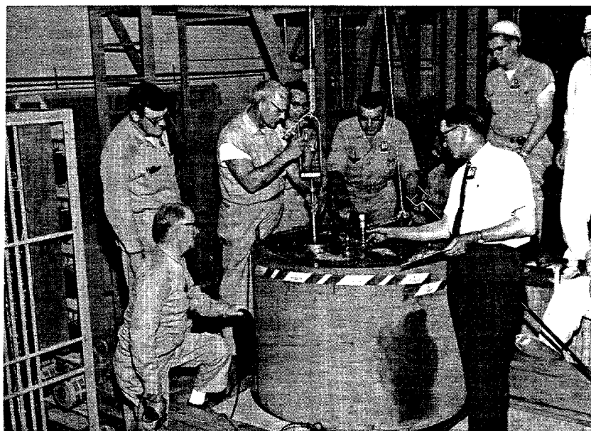
▲ Craftsmen enrolled in the Molten Salt Reactor Experiment training class learn to perform remote maintenance on the reactor. The men are practicing the use of long-handled tools through thick shielding. The instructor for this phase of the training is W. D. Todd, P&E Division. Trainees (left to right) are C. E. Hollifield, J. M. Hackworth, J. T. Maples, C. E. Fritz C. J. Houser, C. E. Mashburn, J. Keeney, A. B. Slusher, and F. M. Barnes, all P&E personnel. (Source: The News, April 21, 1967.)
