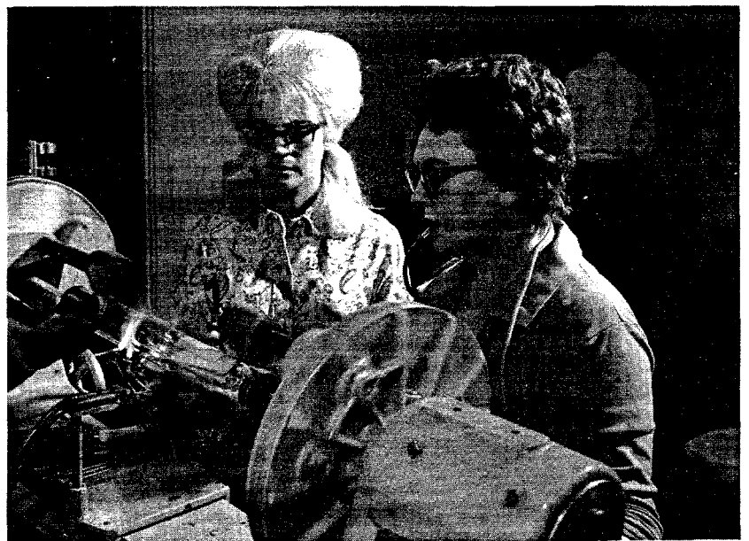
▲ Plater. R. W. Ormsby applying silver plating to Nevada HENRE, or High Energy Neutron Reactions Experiment, target in Plating Shop (1967).
