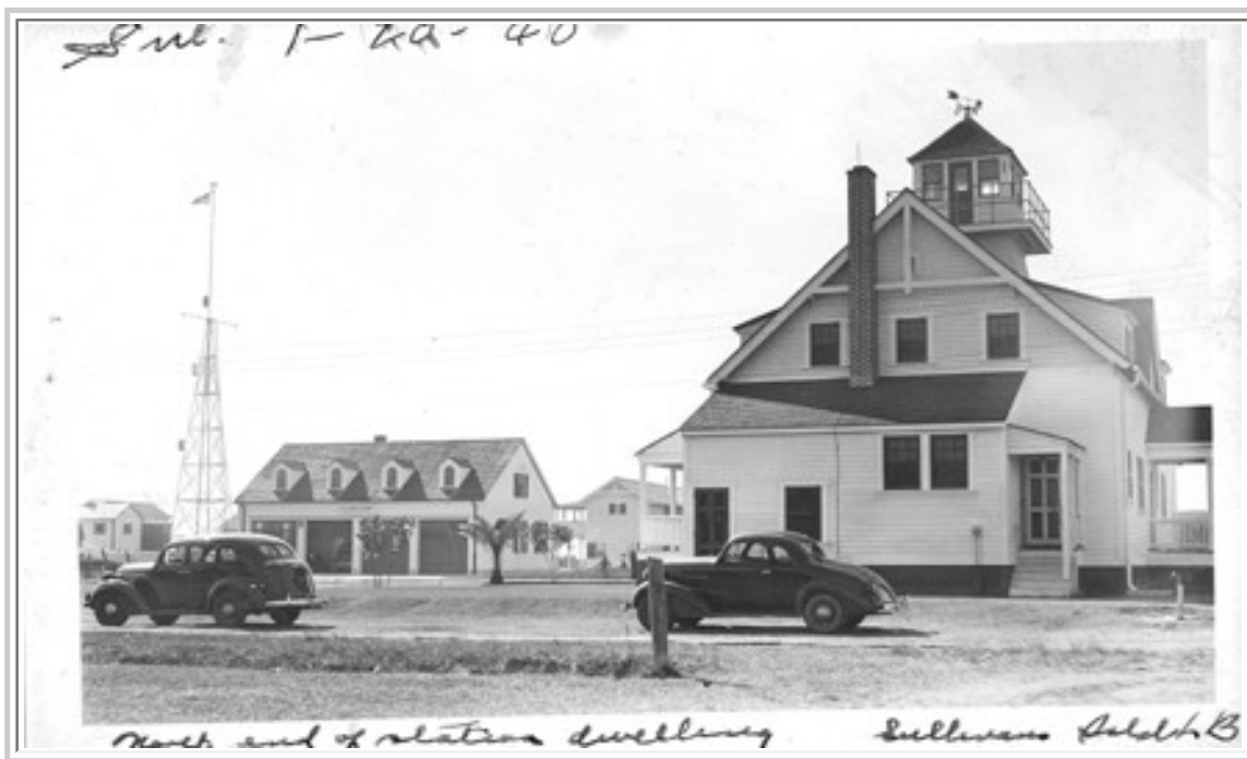
Original photo caption: "North end of station dwelling [;] Sullivan's Isld LB Sul. 1-20-40"; photo dated 20 January 1940; no photo number; photographer unknown.
