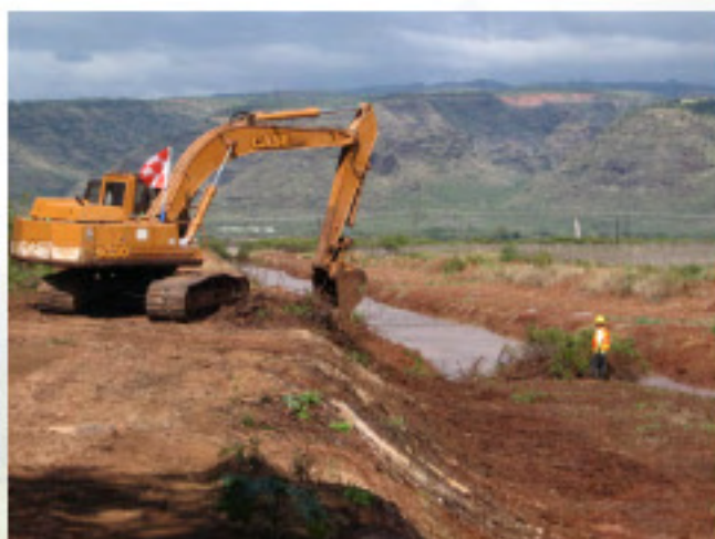
Dredging a drainage canal in Kekaha
