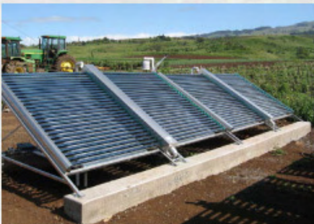
Solar Water Pasteurization panels at Kula Ag Park in Maui
