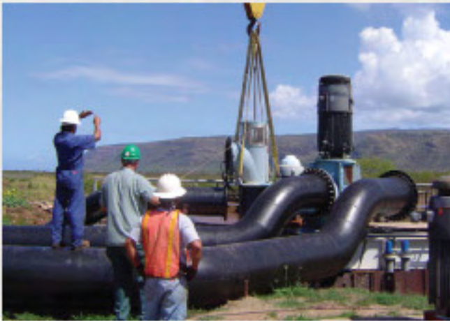
Reinstalling a pump at Kapaehaona pumping station in Kapaehaona
