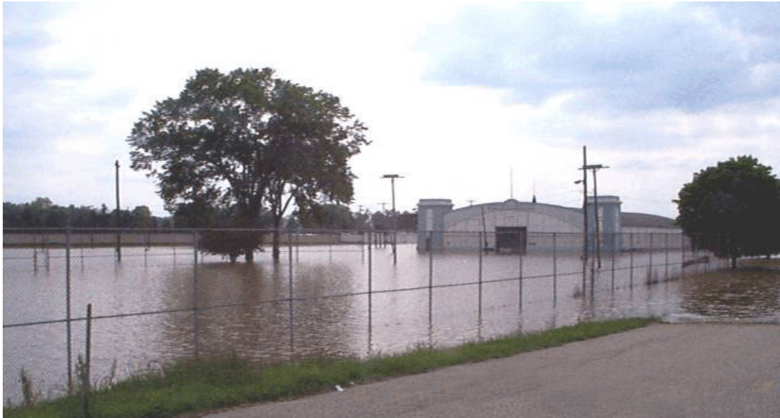
Mississippi River flooding Municipal Airport at 35.5 feet on 2/15/1998.
