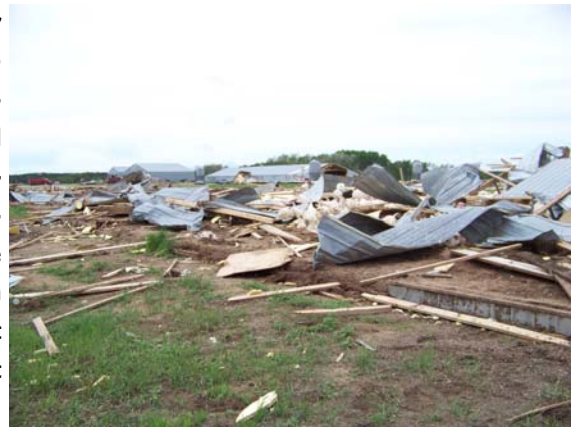
Turkey barns destroyed near the Wadena/Hubbard County line.
