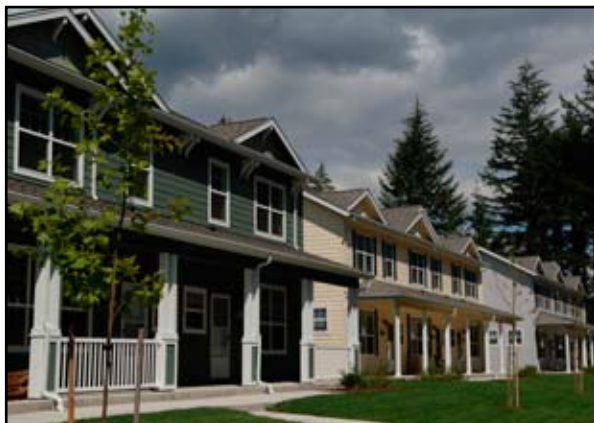
A far cry from military base housing of the past, these modular homes built in Silverton and located at Fort Lewis, Washington, offer functionality and style for soldiers and their families.
