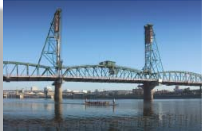
Hawthorne bridge, Portland © Photographer: Dennis Neffendorf | Agency: Dreamstime.com
