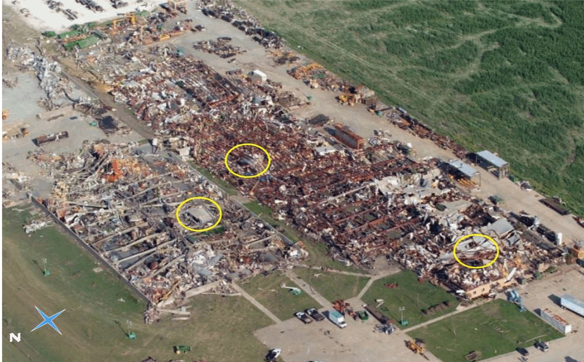
Figure 3. Overhead picture of the damage at the Parsons Company, looking southeast. The yellow circles indicate the locations of the storm shelters. The center of the 0.4 KM wide tornado tracked through the building in the lower left of the picture. Photo courtesy of the Peoria Journal-Star.
