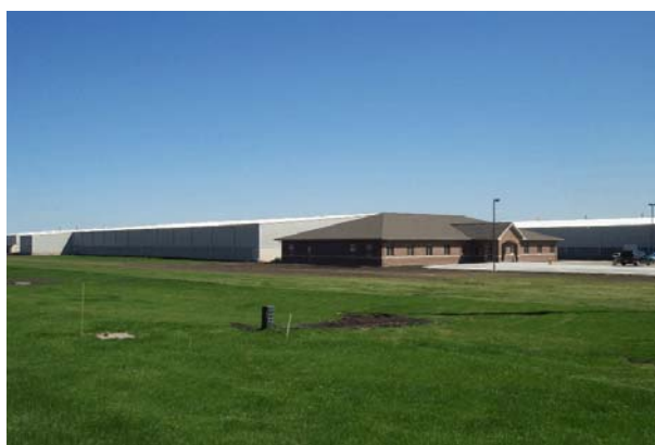
Figure 5. The “new” Parsons facility - April 2005, looking southeast. Photo by NWS.
