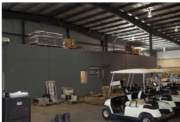
Figure 6. Two side-by-side, concrete and steel reinforced storm shelters in the new Parsons facility. Photo by NWS.
