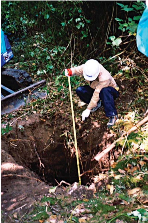
Soil sampling in a test pit at Ellisport Creek site.
