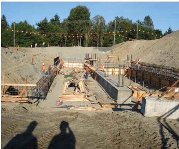
The new First Northeast transfer station under construction.
