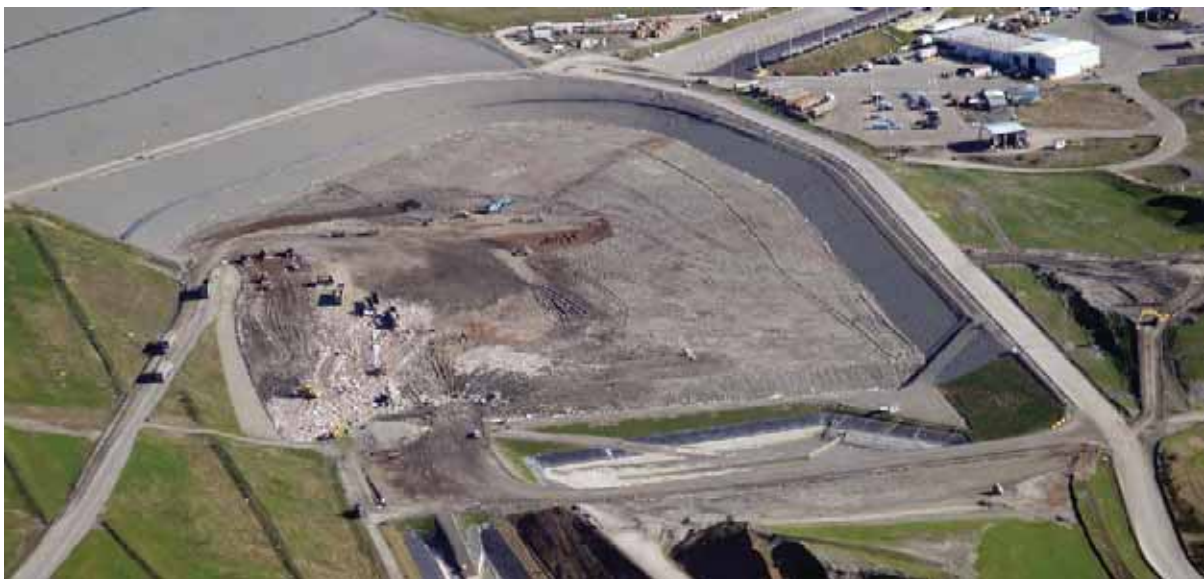
Recently completed Area 6 in the Cedar Hills Regional Landfill.
