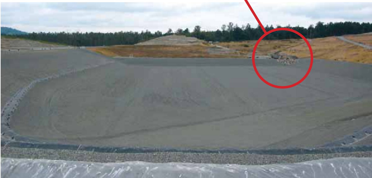
First trucks unloading at newly completed Area 6 at the Cedar Hills Regional Landfill.
