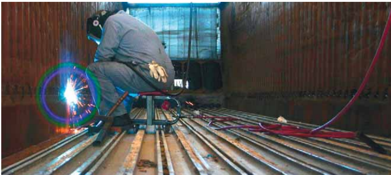
New walking floors being welded into existing trailers.
