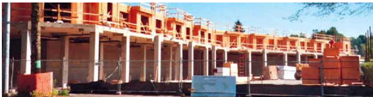
Construction at Rainier Court after cleanup.
