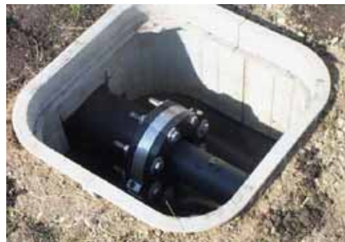
Figure 12. Expansion/Contraction Coupler
