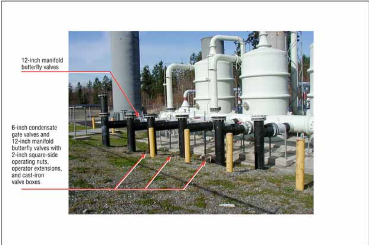
Figure 8. Cyclonic Knockouts at the North Flare Station
