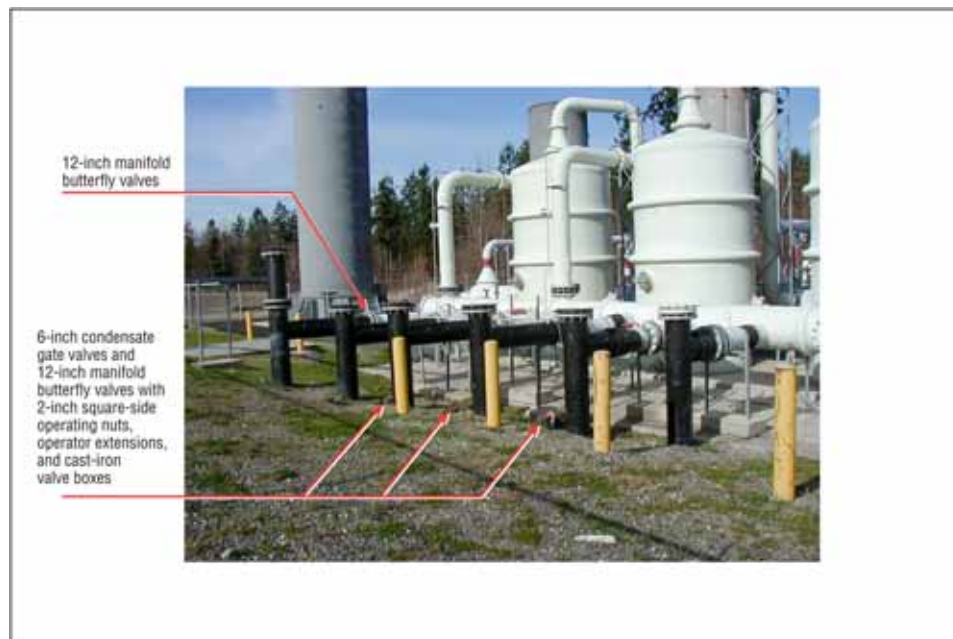
Figure 15. Cyclonic Knockouts at the North Flare Station
