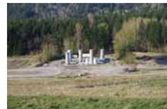
40-foot-high gas flares with buffer zone trees in background
