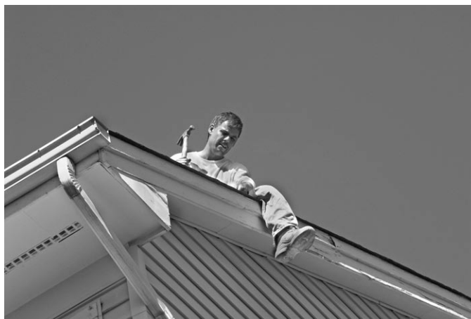
Most residential steep-slope roofs are covered with shingles.
