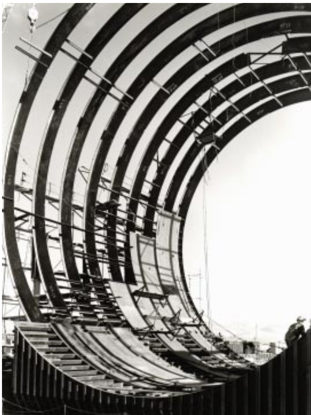
Figure 1. The first big project at the Livermore site began in 1951, before the laboratory itself was approved. This photo shows the prototype vacuum chamber for the so-called Materials Testing Accelerator under construction. Once development was completed, the full mile-long linear accelerator was constructed near St. Louis.
