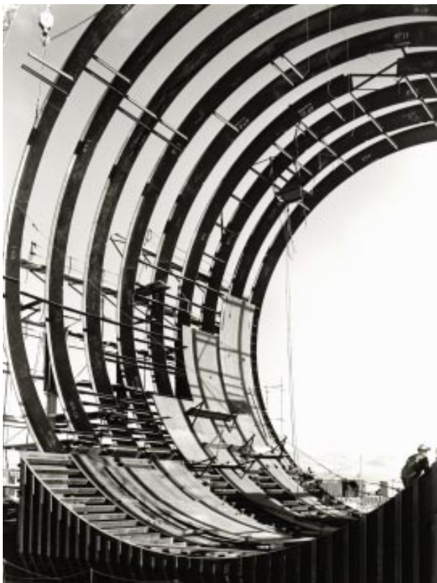
Figure 1. The first big project at the Livermore site began in 1951, before the laboratory itself was approved. This photo shows the prototype vacuum chamber for the so-called Materials Testing Accelerator under construction. Once development was completed, the full mile-long linear accelerator was constructed near St. Louis.
