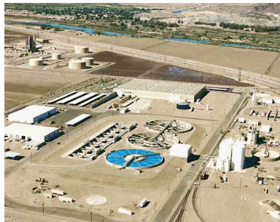
Figure 9 – Aerial Photo of Yuma Desalting Plant.
