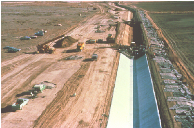
Figure 12 - Photo of Canal Lining.
