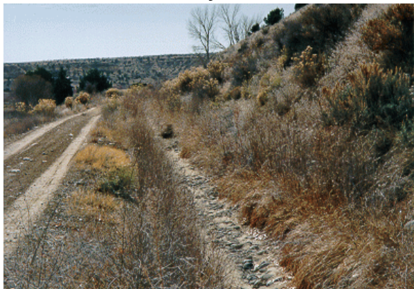
Figure 19 - Unimproved Canal at Hammond Project.
