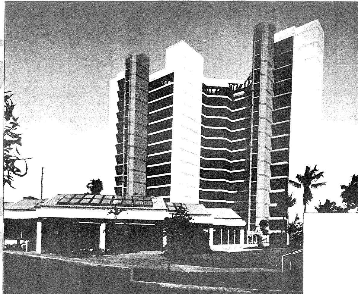
E.1&2 USS Arizona Hall, 1984. This US Navy highrise barracks is cooled by natural ventilation. Architect: Media 5 Limited. Energy Consultant: TRB Hawaii. Photograph: Angie Salbosa.
