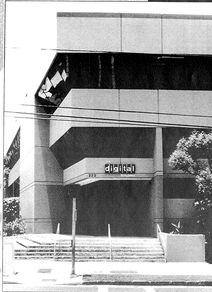
B.1 The Digital Equipment Corporation Building, 1979. The upper floors step out to shade the glass below. Architects: Anderson Reinhardt. Photo: Max Raksasat.
