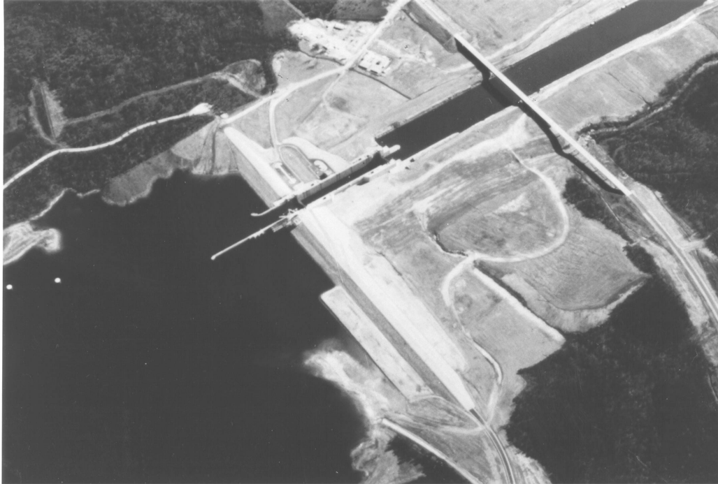
Figure 12. Bay Springs Lock, Tennessee-Tombigbee Waterway, illustrates a high-lift lock that bypasses the river regulation and flood control facilities
