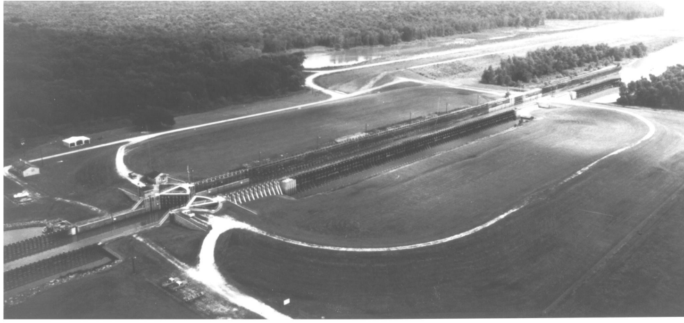
Figure 14. Vermilion, on the Gulf Intercoastal Waterway, Louisiana, is a low-lift navigation project
