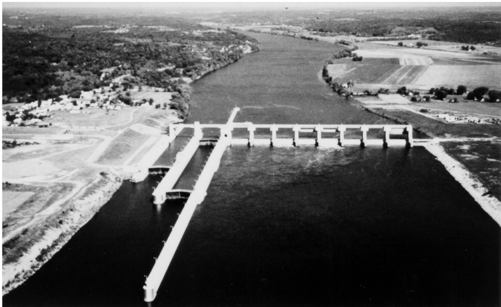
Figure 13. Belleville Lock and Dam on the Ohio River illustrates a typical medium-lift navigation project
