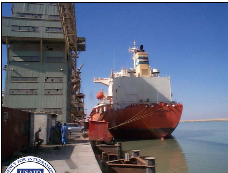
The MV Banastar, the first bulk cargo grain ship to arrive at Umm Qasr since the 2003 conflict finished unloading 52,000 tons of grain on November 14, 2003. The newly refurbished grain-receiving facility moved the grain from the ship to dockside silos without major problems. (USAID photo)
