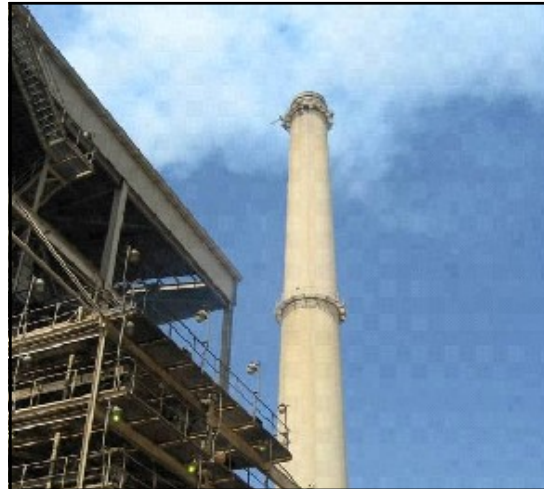
Operating unit at a USAID power plant project in central Iraq
