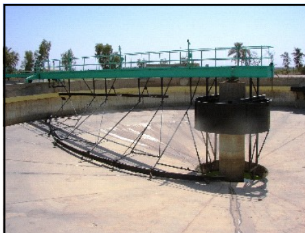
A wastewater treatment facility in central Iraq being rehabilitated by USAID
