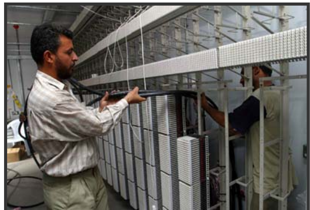
The Al-Mamoun Telephone Exchange where repair work will restore telephone services to approximately 30,000 subscribers. (Photo: Thomas Hartwell)
