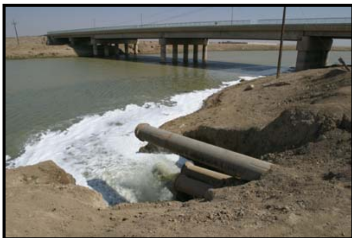
Nasiriyah, Iraq - Raw sewage is dumped into the Euphrates River at Nasiriyah in southern Iraq. Wastewater treatment plants were insufficient before the war, and many were looted in the aftermath. USAID partner RTI is finding solutions for the aging, poorly maintained water and wastewater infrastructures. (Photo: Thomas Hartwell)
