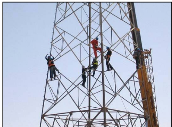
Erecting a tower on the Khor az Zubayr-An Nasiriyah 400 KV line.
