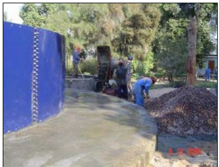
Ongoing work at a Basrah thermal power plant.
