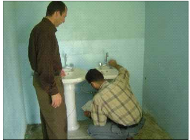
NGO engineers monitoring the rehabilitation of school bathrooms
