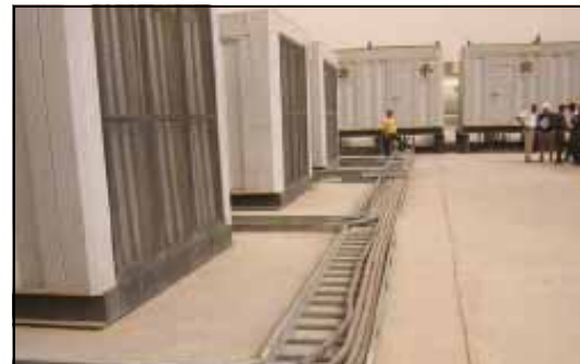
Laying power cables between generators.
