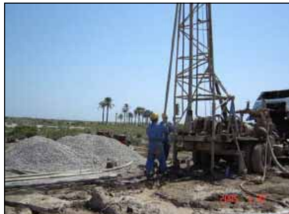
Well-drilling has begun at 74 sites in rural areas.
