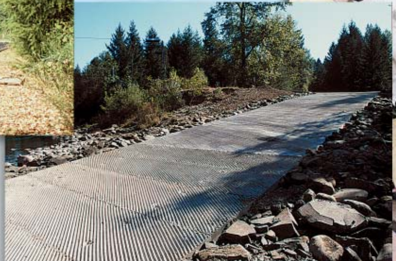
▶ Better parking and traffic flow, and a solid, self-cleaning concrete ramp are ready for rafters this spring.
