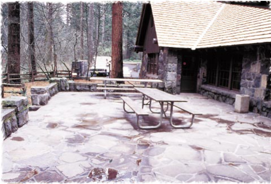
Patio masonry work done in 1999 salvaged much of the original flagstone rock from the early days of the park.
