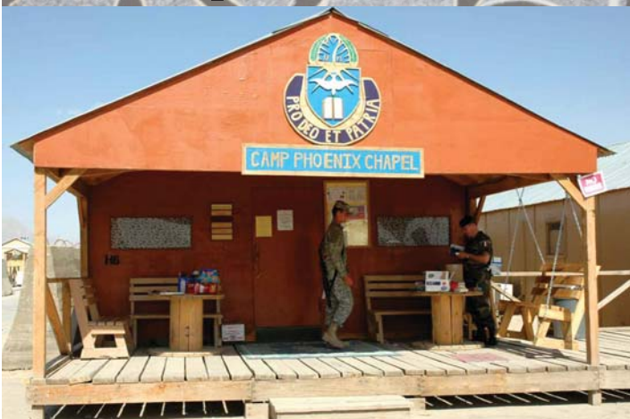
The Camp Phoenix Chapel before remodeling.
