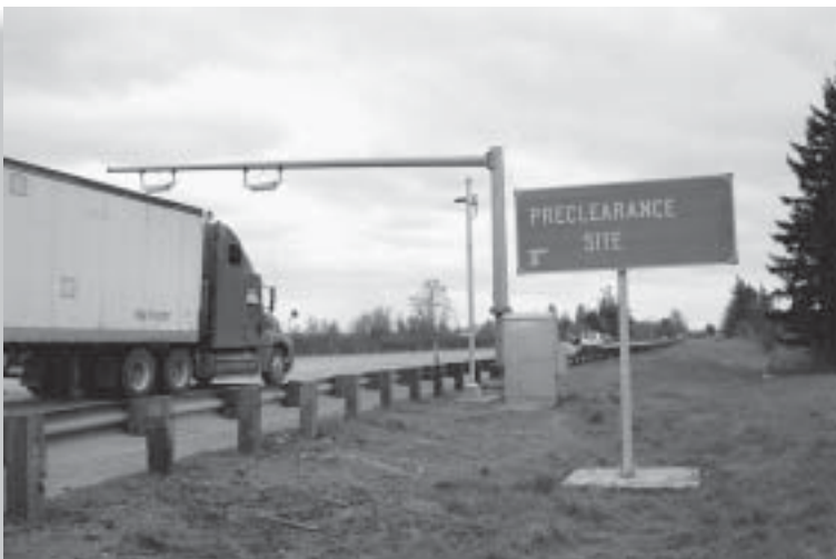
Oregon Green Light preclearance systems, like this one at the Woodburn Port of Entry on southbound Interstate 5, have allowed trucks to avoid stopping at weigh stations more than three million times since January 1999.
