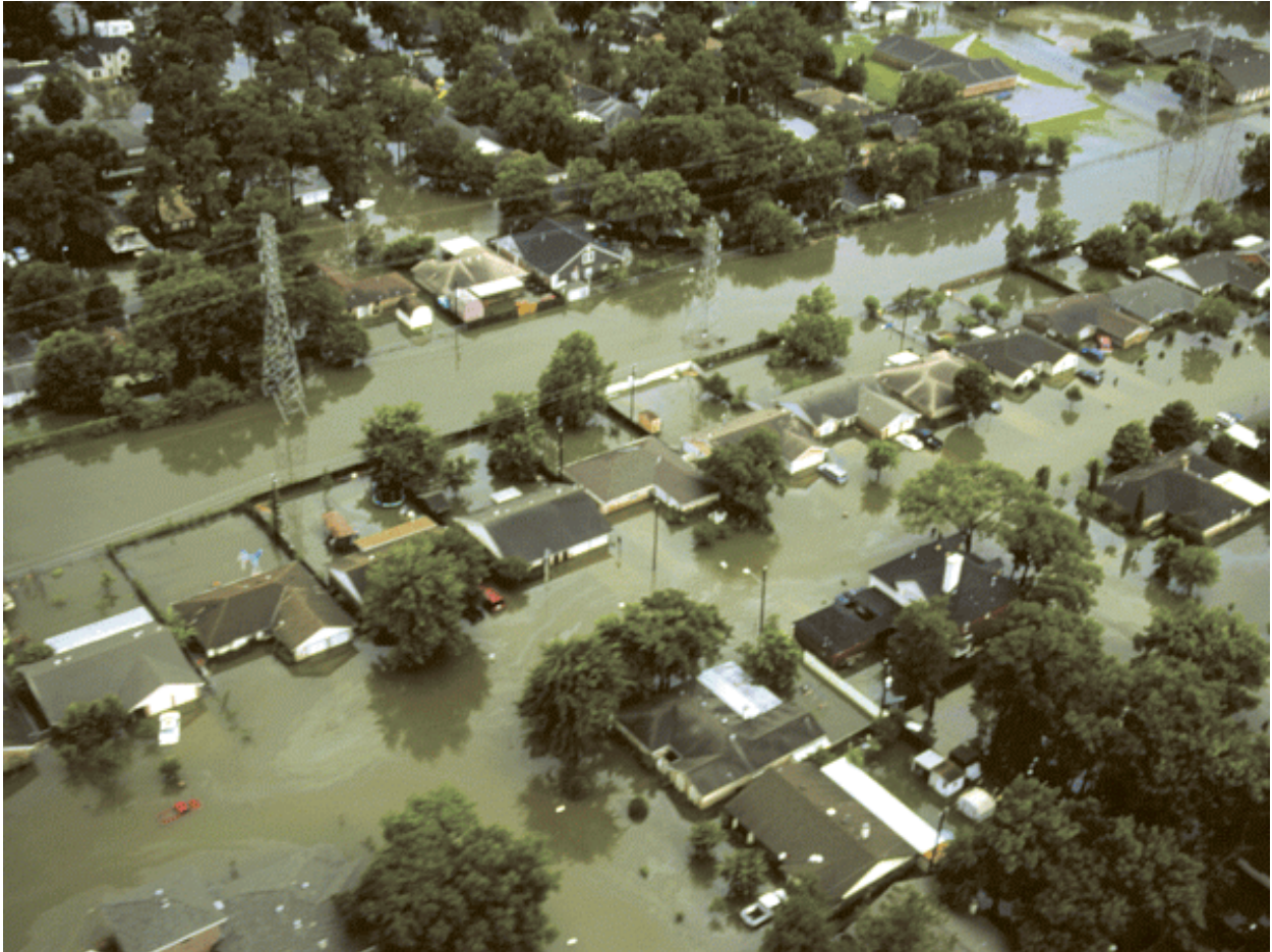
Neighborhood flooding near Interstate 10, Houston, Texas. (Courtesy of Harris County Flood Control District/Steve Fitzgerald)
