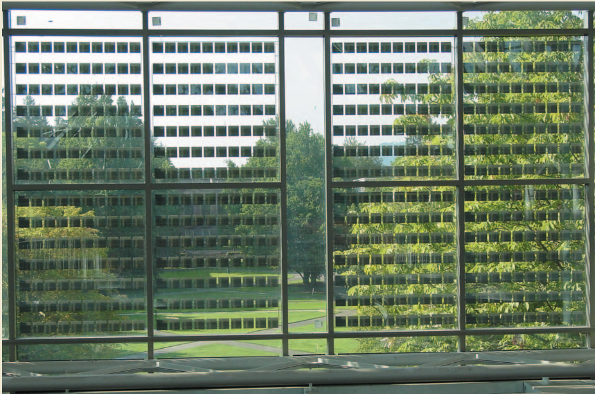
At left, solar panels greet the students at the front of the Lillis Building. The panels provide about 6 percent of the electricity for the whole building. Below, theater seating was planned for the largest lecture hall in the Lillis Building. Each seat has a power source for laptop computers. Photos courtesy of the Oregon Department of Energy.
