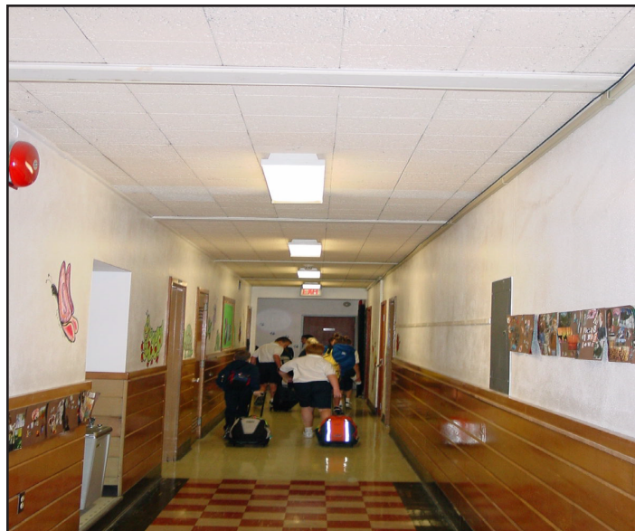
The hallways at St. John the Baptist school use to be dark. With more energy-efficient lighting, they are brighter.
