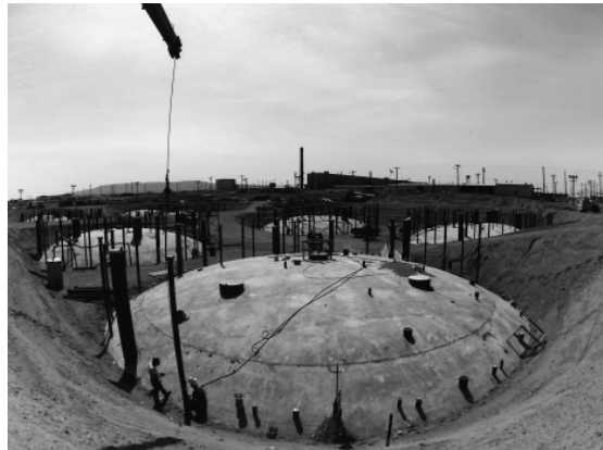
Hanford Tank Under Construction
