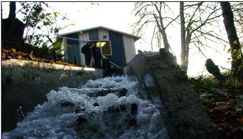
Water tumbles down into Baker Creek after it generates electricity. It is aerated before it enters the creek.
