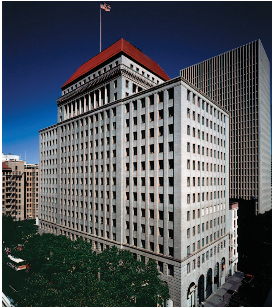
One of Portland's historic skyscrapers, the Public Service Building also had lofty energy bills before a recent renovation reduced energy costs by some $160,000 a year. Photo courtesy of the Downtown Development Group.
